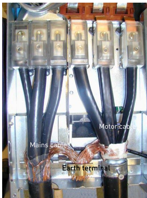
Figure 6-18. Cable installation in Vacon NXS/P, FR8
