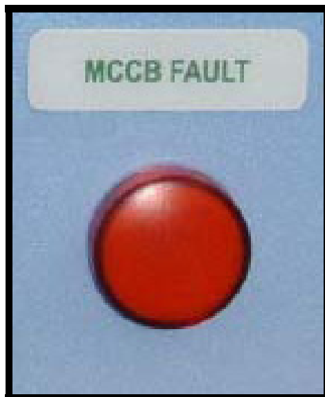
Figure 29. MCCB FAULT indicator
