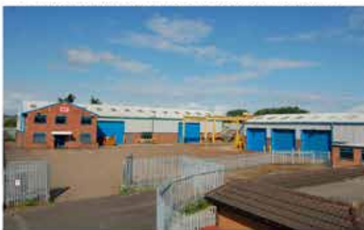
Head office and specials division
