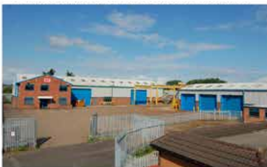
Head office and specials division
