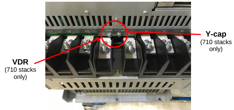
Bottom Terminal Area
