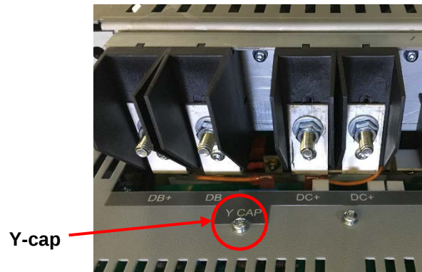
Top Terminal Area
